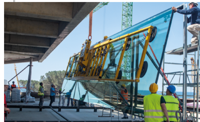
Vacuum suction system VSG 6000 KMH with 15 m pane
