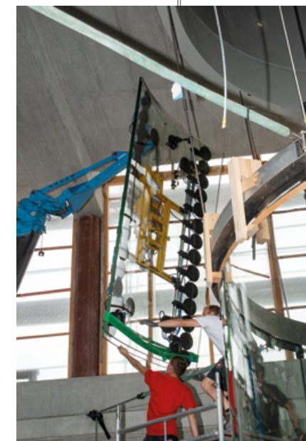
The MRK 144.0 S mounting crane and the VSG 1000 KR vacuum suction system used to glaze the flight chamber
