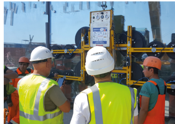
On-site instruction: the VSG 1500 KH vacuum suction system
