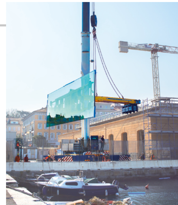
Transportation of pane over 40 m across the port
