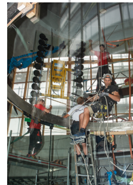
The MRK 144.0 S mounting crane and the VSG 1000 KR vacuum suction system used to glaze the flight chamber
