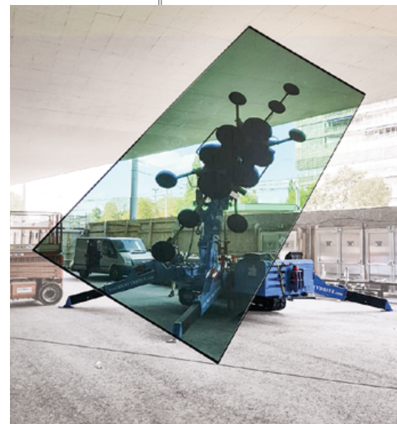
Glass mounting under an overhang with the VSGU 1500 KMH
