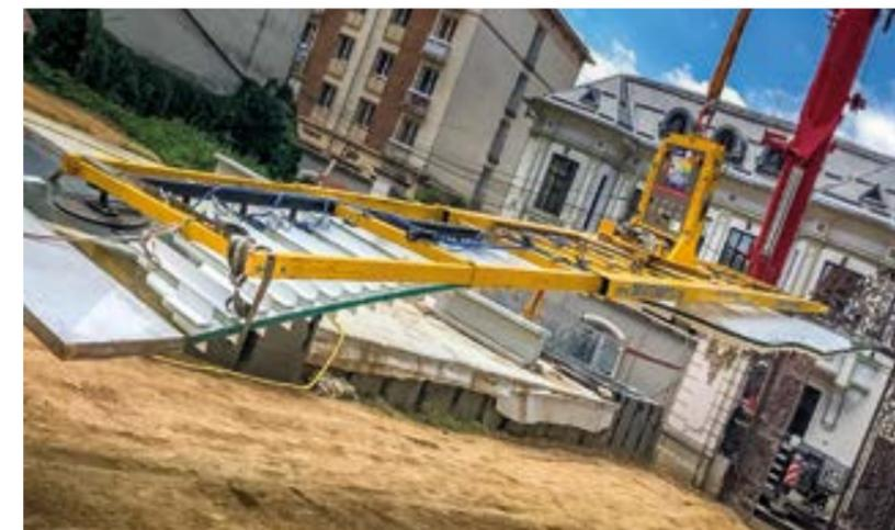
The Heavydrive system transports 12.5 metre high designer pane with wavy edges. Image rights: montec-gmbh.de
