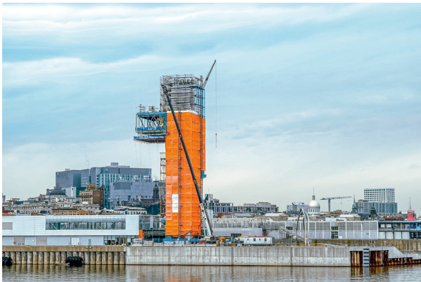
Montarea sticlei Heavydrive la Tour du Grand Quai din Montréal QC (Canada)
